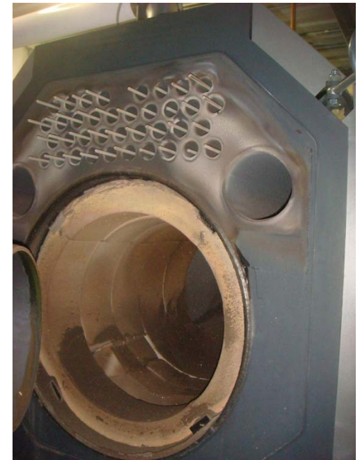
Secondary Chamber Burns Gas Heat Exchanged to Water – Flue Gas Recycled
